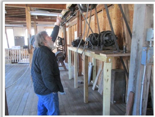
1920's Line Shafting and Motors
